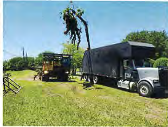
Debris removal from Oyster Creek
