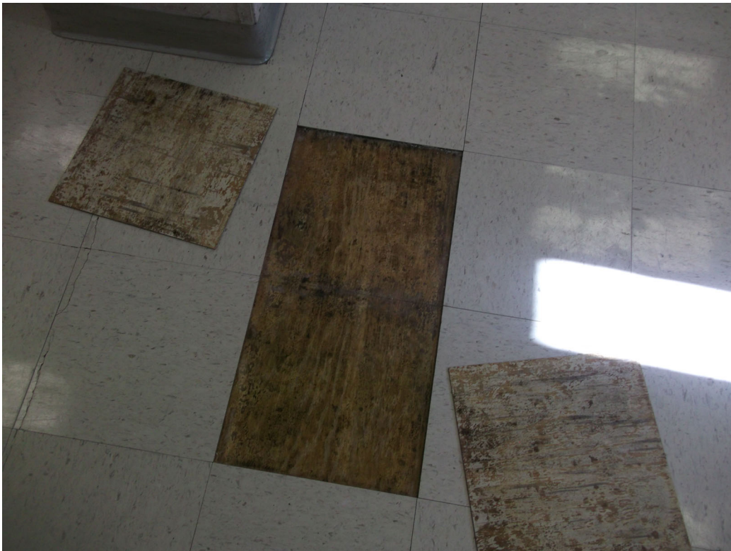
PHOTO 4 – 11/29/2022 PHOTO SHOWING MOLD-IMPACTED PLYWOOD SUBFLOOR IN THE SOUTH CENTER SIDE OF THE MAIN ACTIVITY ROOM.
