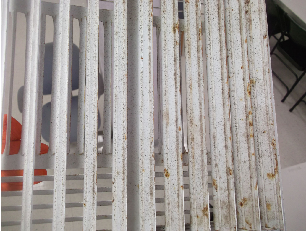
PHOTO 177 – 11/29/2022 PHOTO SHOWING DUST AND CORROSION ON THE METAL AIR DIFFUSER VENTS.
