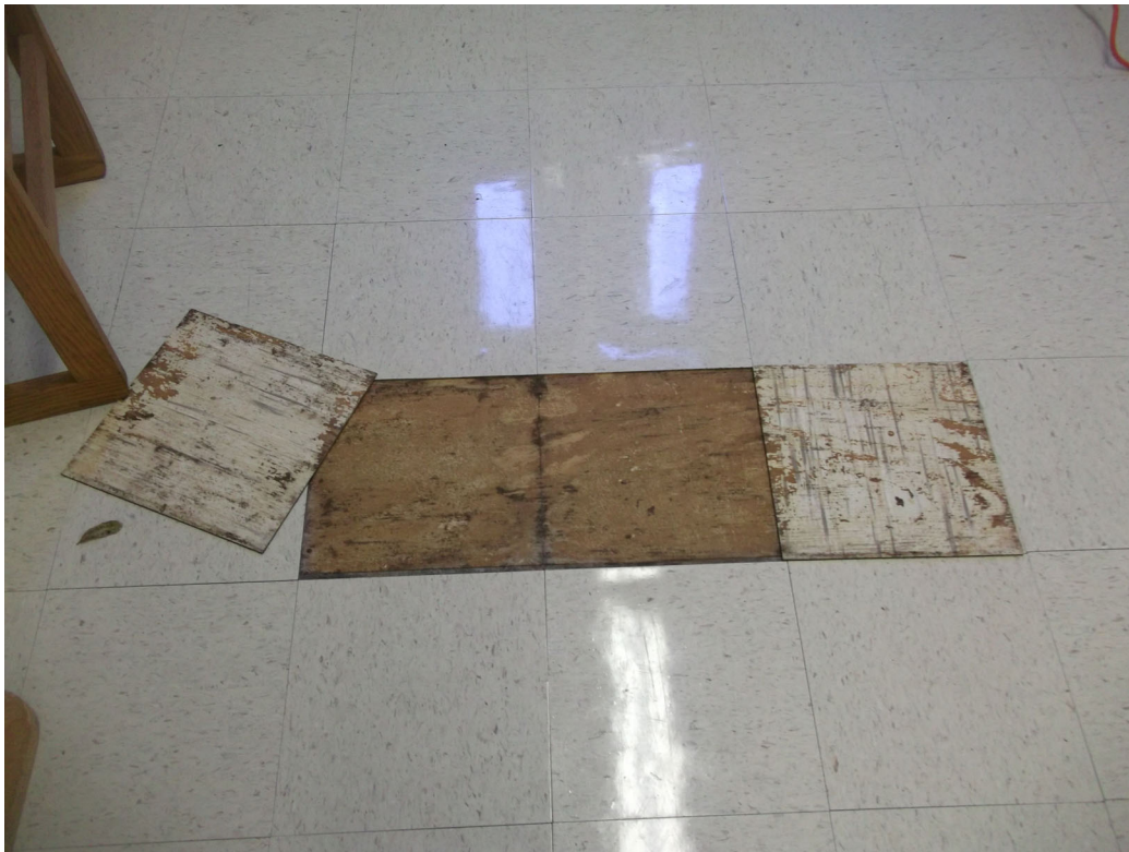
PHOTO 7 – 11/29/2022 PHOTO SHOWING MOLD-IMPACTED PLYWOOD SUBFLOOR IN THE LOBBY.
