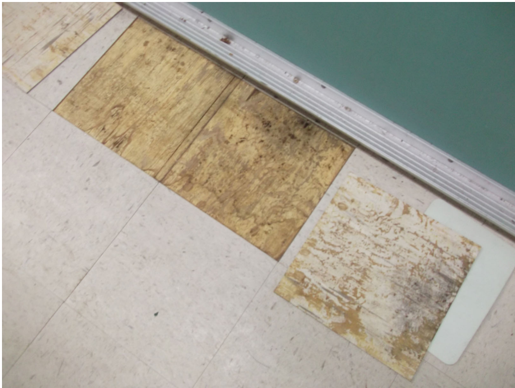
PHOTO 5 – 11/29/2022 PHOTO SHOWING MOLD-IMPACTED PLYWOOD SUBFLOOR IN THE STOREROOM.
