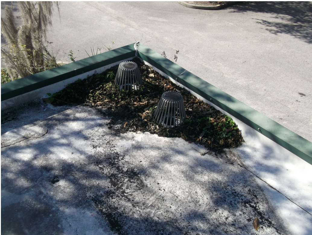
PHOTO 16 – 11/29/2022 PHOTO SHOWING THE BLOCKED DRAINS AT THE SOUTHWEST CORNER OF THE ROOF.
