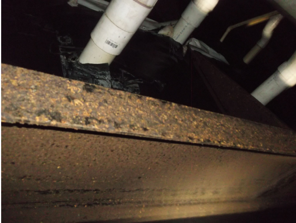
PHOTO 189 – 11/29/2022 PHOTO SHOWING OPENINGS IN THE MOISTURE BARRIER UNDER THE NORTH MODULAR SECTION OF THE BUILDING.
