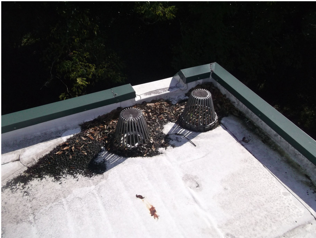
PHOTO 14 – 11/29/2022 PHOTO SHOWING THE BLOCKED DRAINS AT THE SOUTHEAST CORNER OF THE ROOF.
