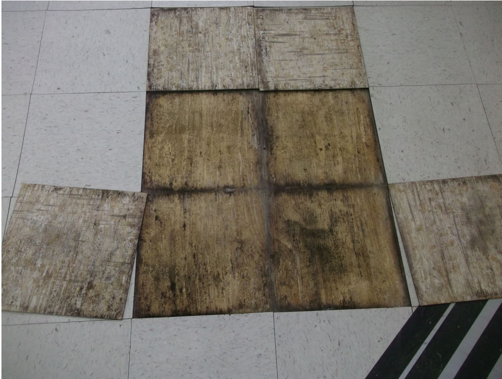
PHOTO 3 – 11/29/2022 PHOTO SHOWING MOLD-IMPACTED PLYWOOD SUBFLOOR IN THE SOUTHEAST SIDE OF THE MAIN ACTIVITY ROOM.
