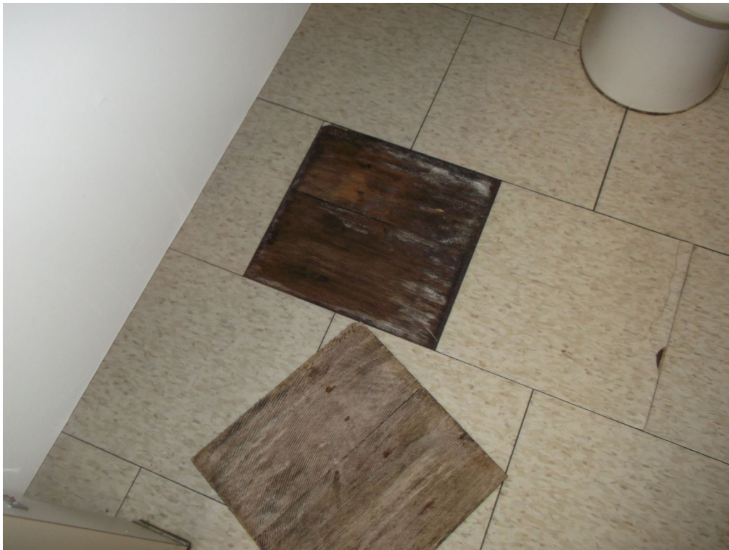
PHOTO 9 – 11/29/2022 PHOTO SHOWING MOLD-IMPACTED PLYWOOD SUBFLOOR IN THE WOMEN'S RESTROOM.
