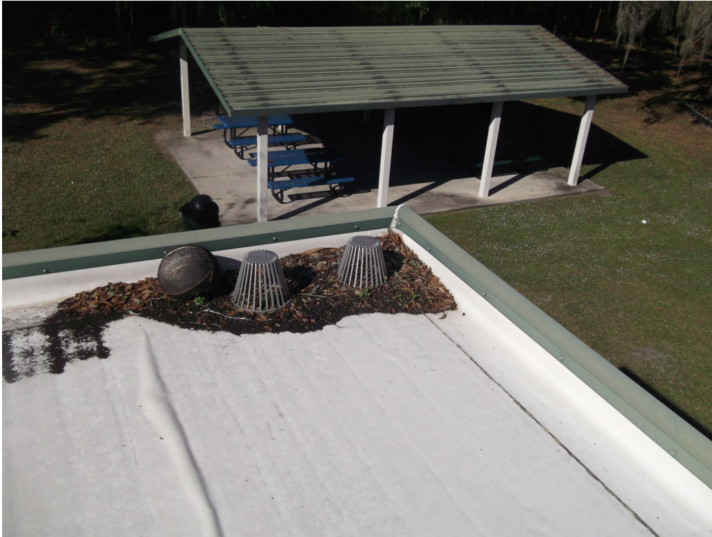
PHOTO 15 – 11/29/2022 PHOTO SHOWING THE BLOCKED DRAINS AT THE NORTHWEST CORNER OF THE ROOF.
