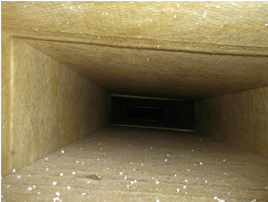
PHOTO 18 – 11/29/2022 PHOTO SHOWING DUST AND DEBRIS BUILD-UP INSIDE THE FIBERGLASS DUCTWORK.
