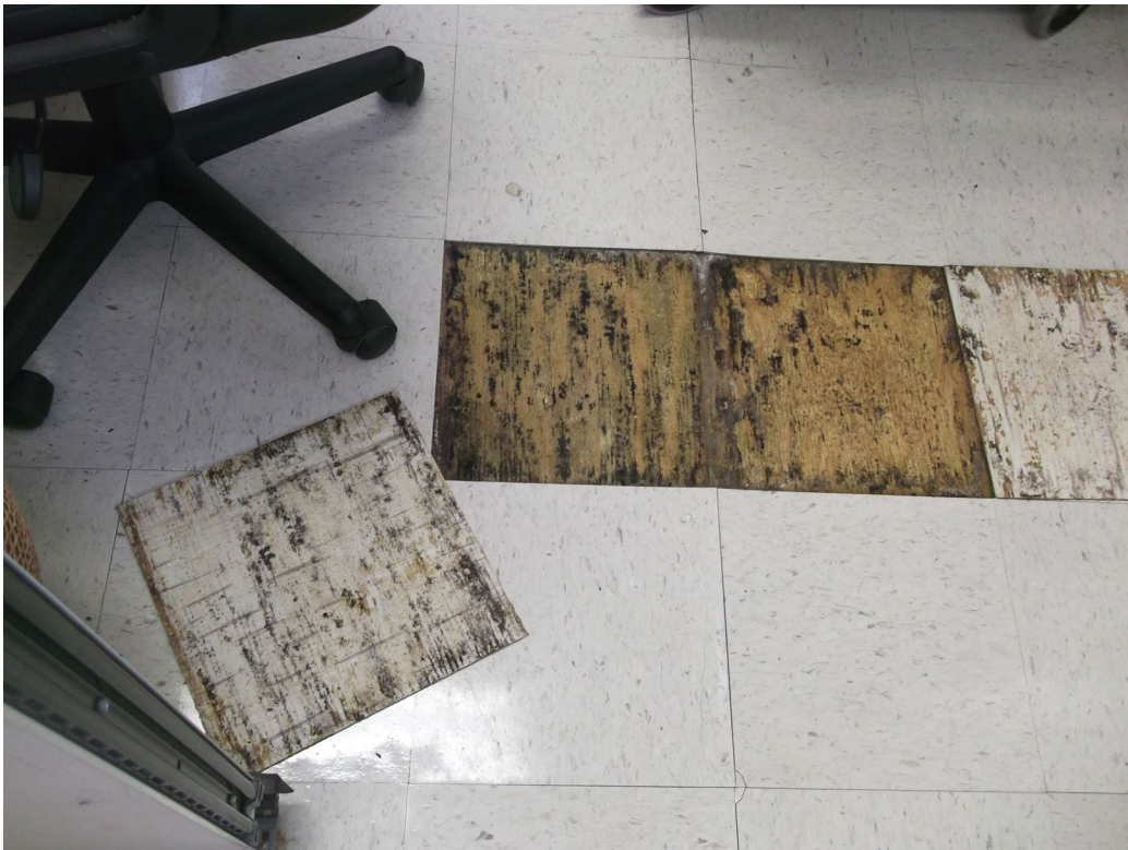
PHOTO 2 – 11/29/2022 PHOTO SHOWING MOLD-IMPACTED PLYWOOD SUBFLOOR IN THE OFFICE CUBICLE.
