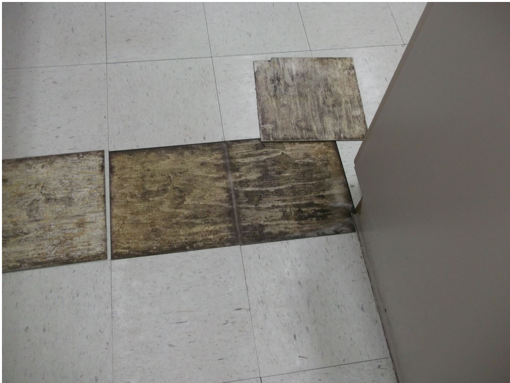
PHOTO 10 – 11/29/2022 PHOTO SHOWING MOLD-IMPACTED PLYWOOD SUBFLOOR IN THE KITCHEN.
