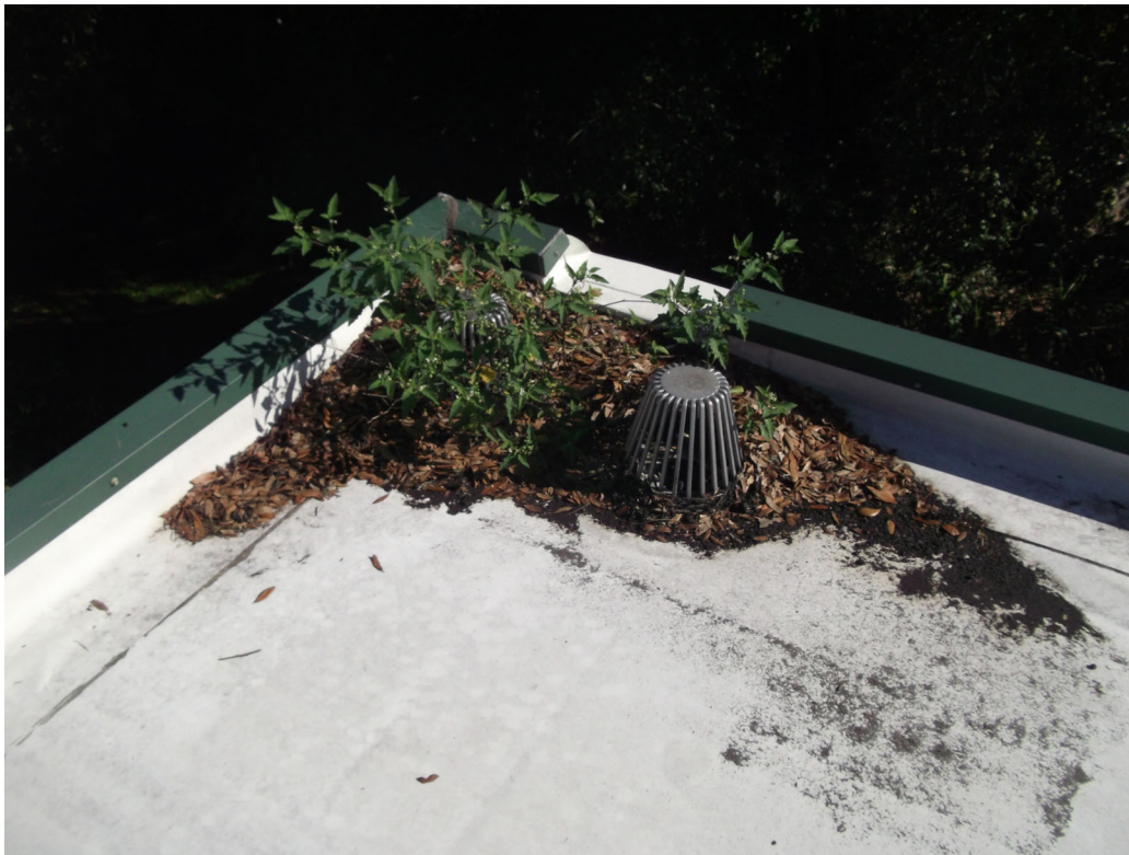
PHOTO 13 – 11/29/2022 PHOTO SHOWING THE BLOCKED DRAINS AT THE NORTHEAST CORNER OF THE ROOF.
