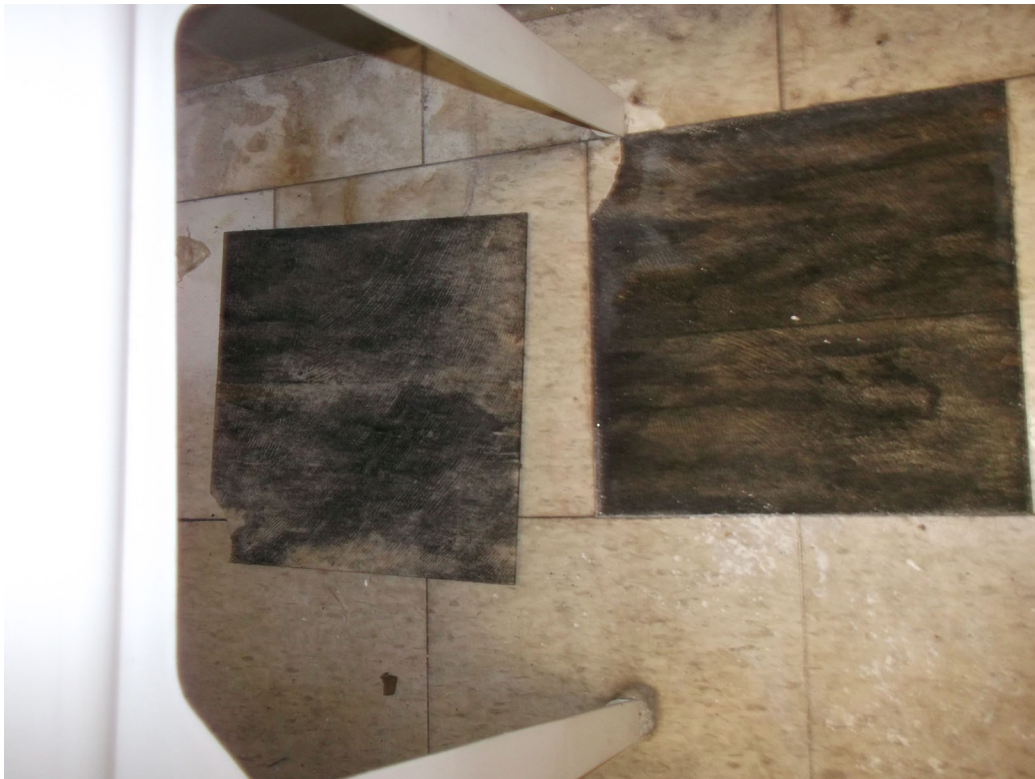
PHOTO 6 – 11/29/2022 PHOTO SHOWING MOLD-IMPACTED PLYWOOD SUBFLOOR IN THE JANITOR'S CLOSET.
