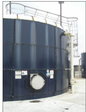
WEST TANK MANWAY AND FILL LINE VIEW
