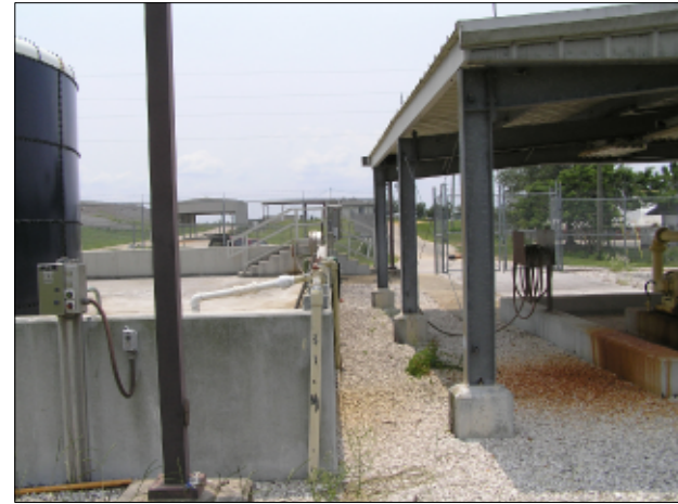
BETWEEN WEST TANK AND PUMP PAVILION SOUTHWARD VIEW B E-1
