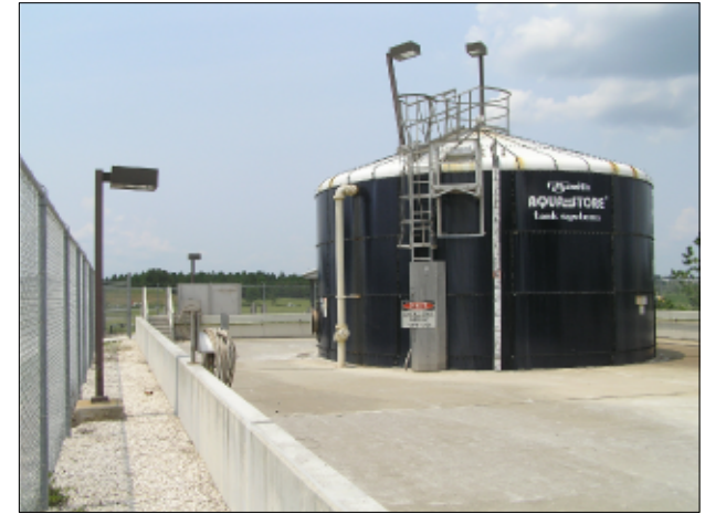
WEST TANK & SECONDARY CONTAINMENT WALL VIEW
