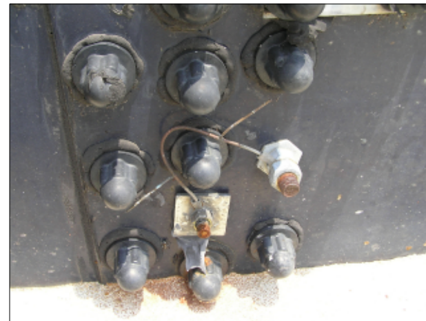
SACRIFICIAL ANODE ASSEMBLY VIEW G E-1
