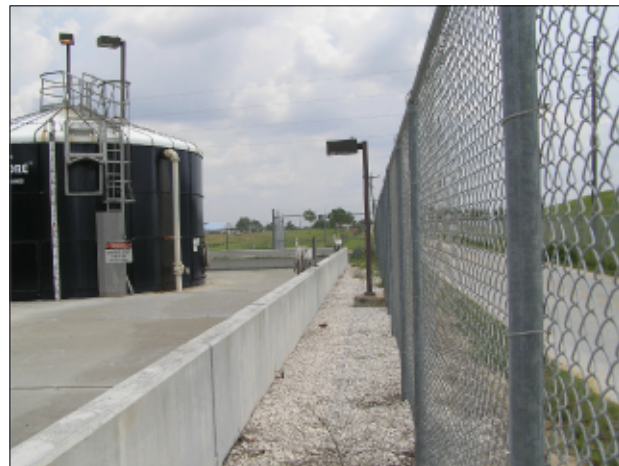
EAST TANK & SECONDARY CONTAINMENT WALL VIEW
