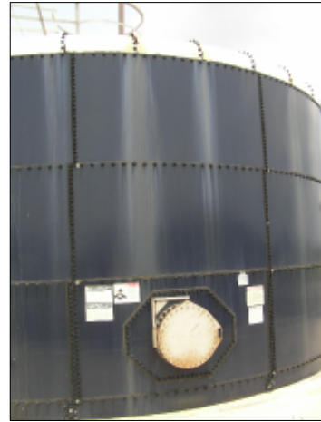
EAST TANK MANWAY VIEW A M-1
