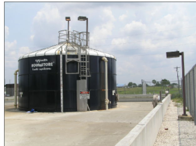
EAST TANK AND SOUTH CONTAINMENT VIEW F E-1
