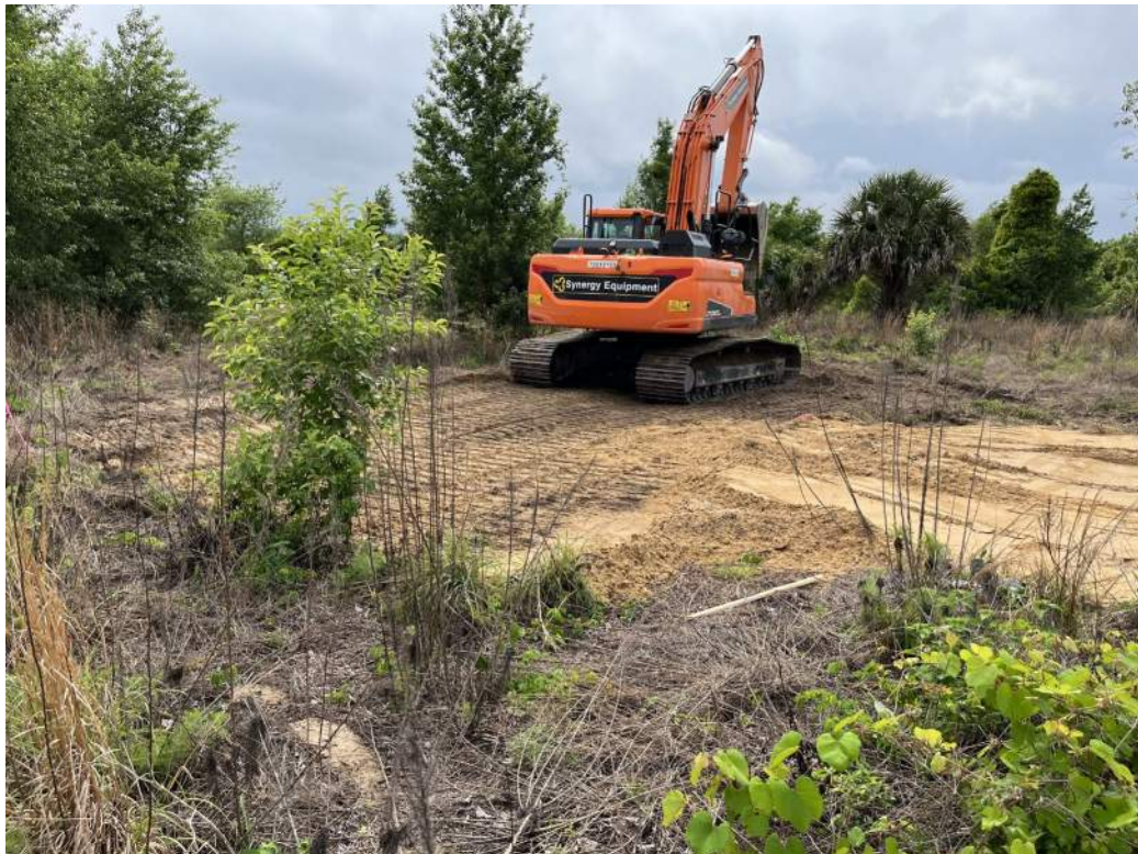
Photo 4: Representative view of the completed ISR area.
