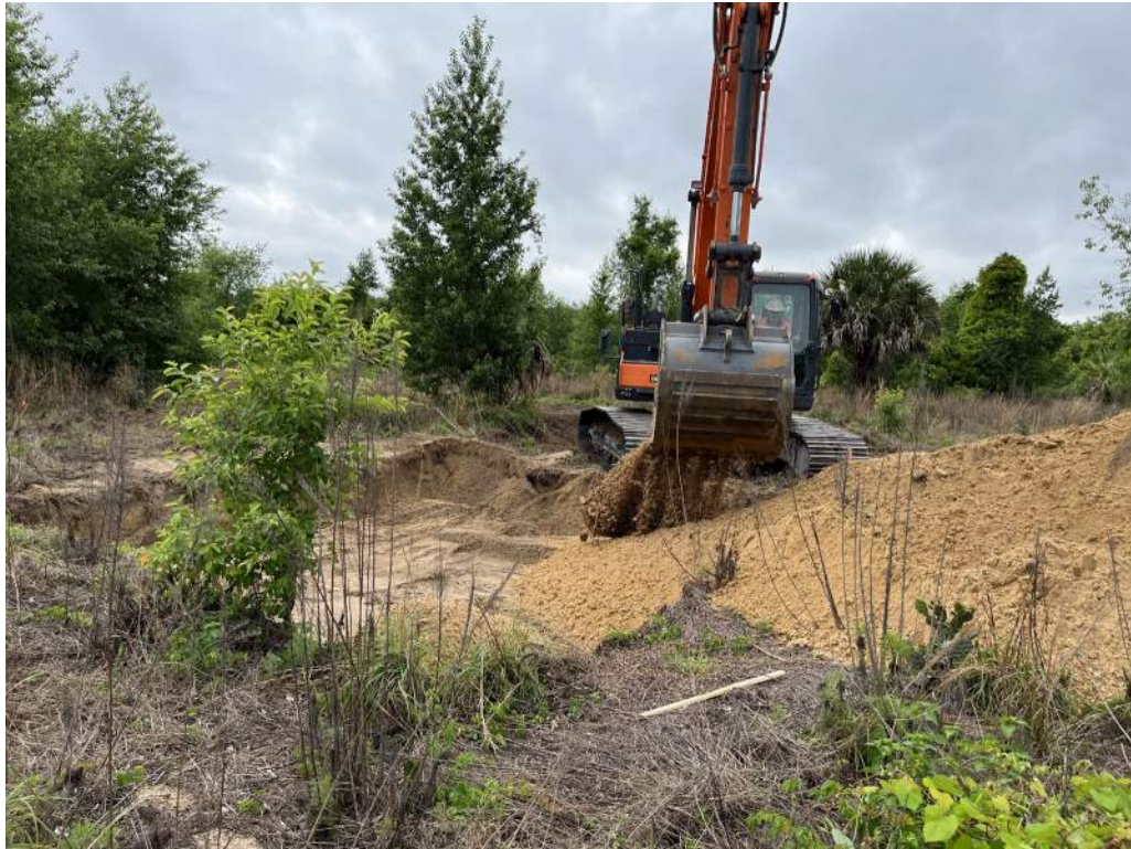
Photo 3: View of backfilling activities within the ISR excavation area.
