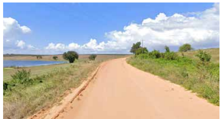
▲ Existing Clay Road
