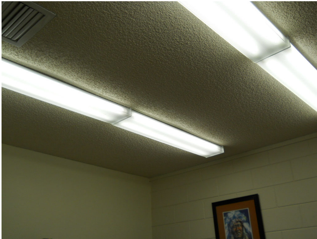
PHOTO 14 – 9/29/21 – INTACT EXPOSED CEILING TREATMENT ROOM 4
