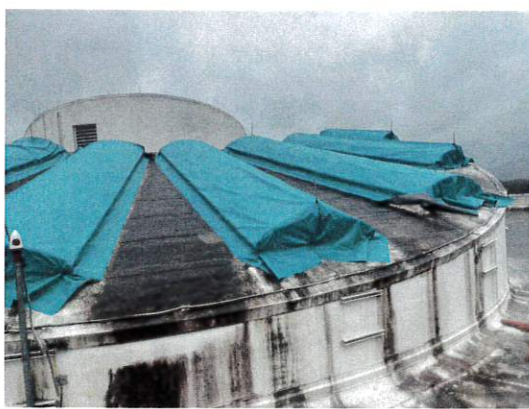
② PHOTOGRAPH OF EXISTING SKYLIGHTS LOOKING NE 1/8" = 1'-0"
