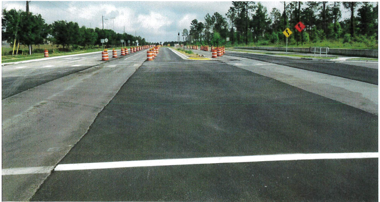
North end of project
