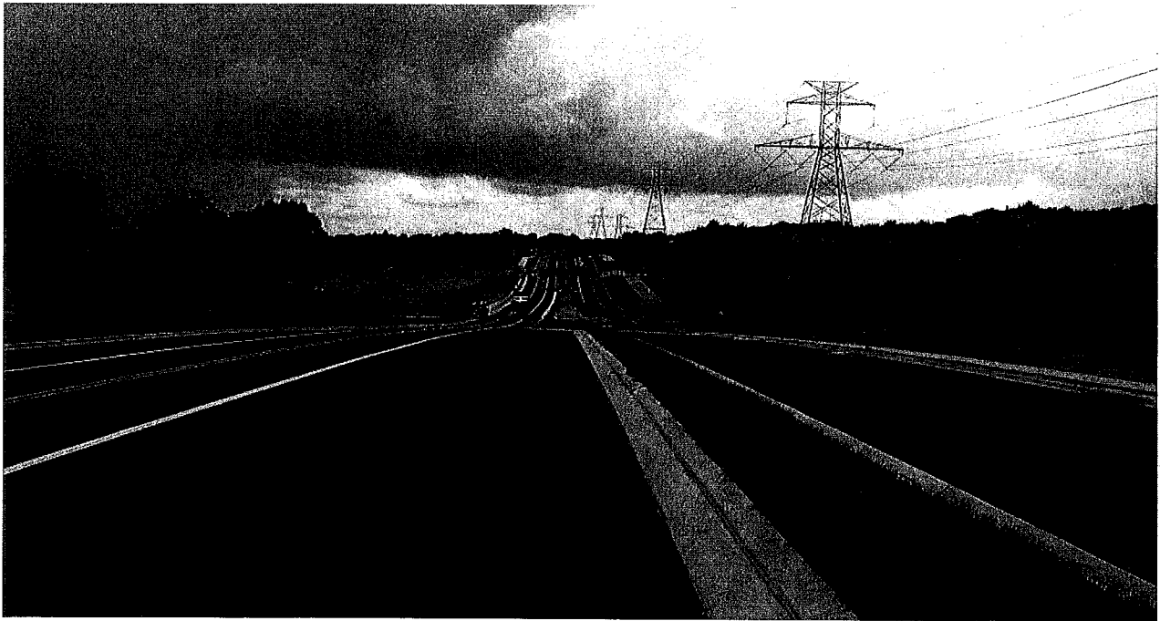
View south from new intersection with West Old Highway 50
