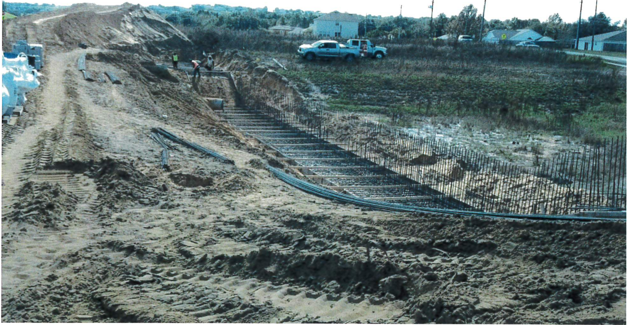
Foundation work near Big Sky Dr
