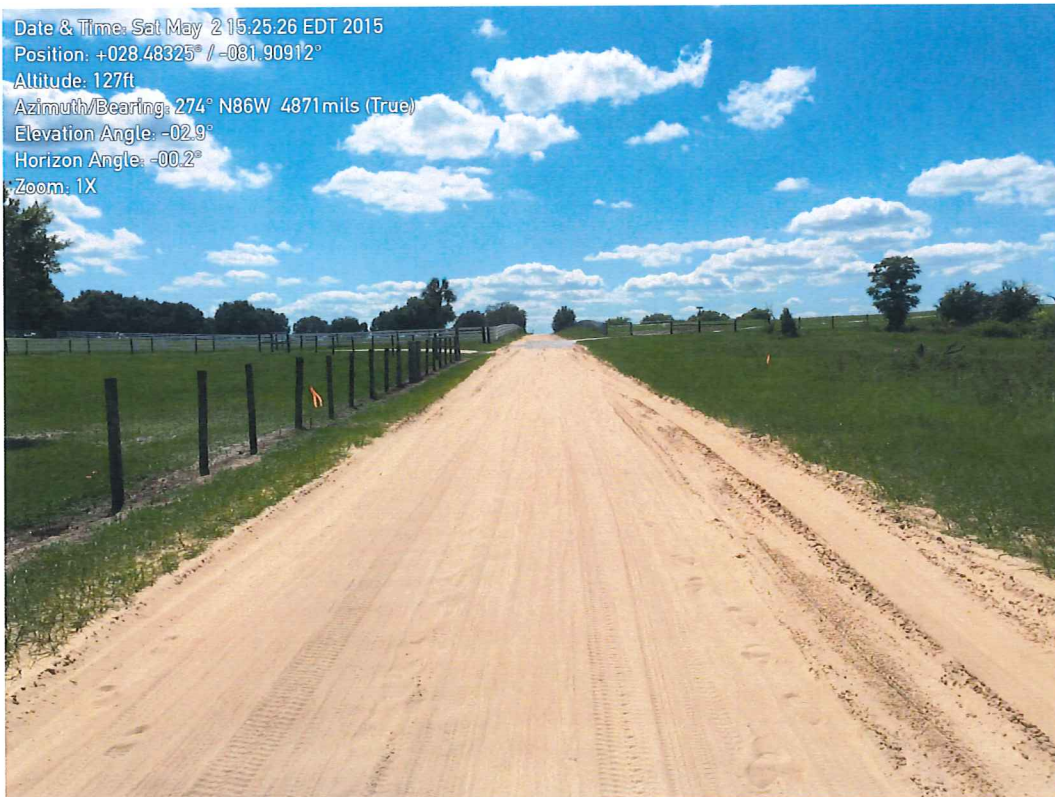
View West (Shady Lane)
