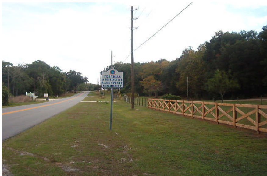
Existing Picture (1) of C.R. 561A Corridor along Ferndale Community
