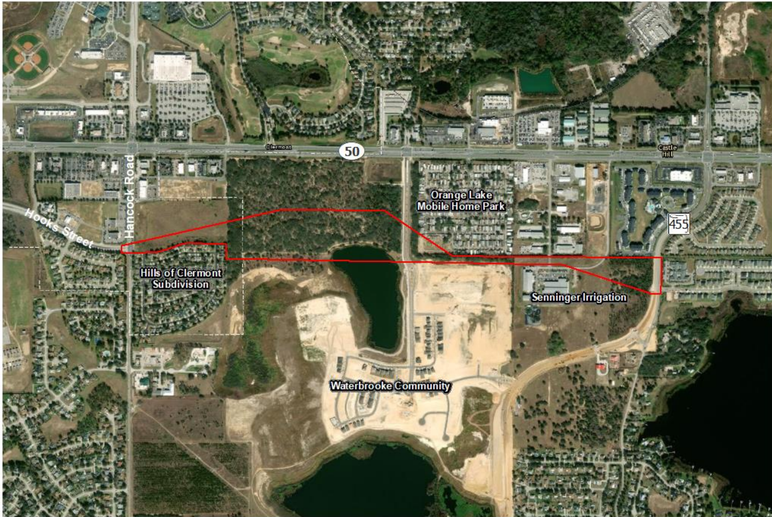
Aerial Photograph Metro Consulting Group, LLC Hooks Street RSQ #20-0906 From Hancock Road to CR 455, Lake County, Florida
