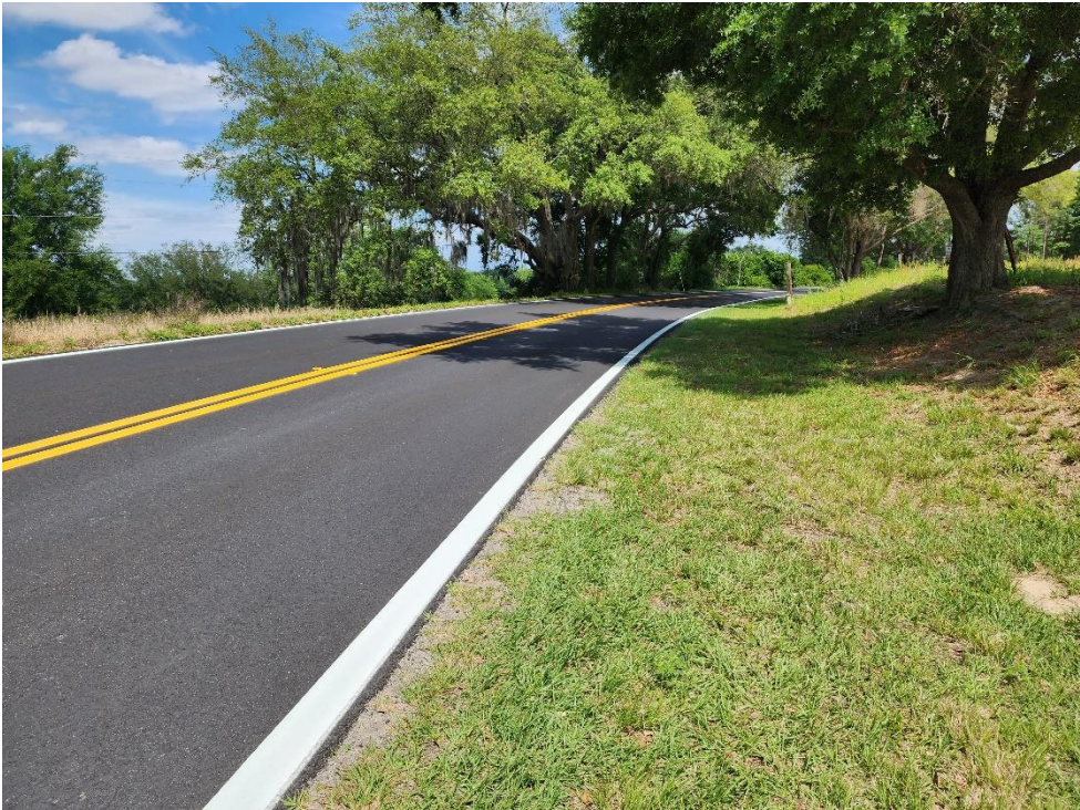
Photo 6 – View of the right-of-way area looking northeast on Lakeshore Drive.
