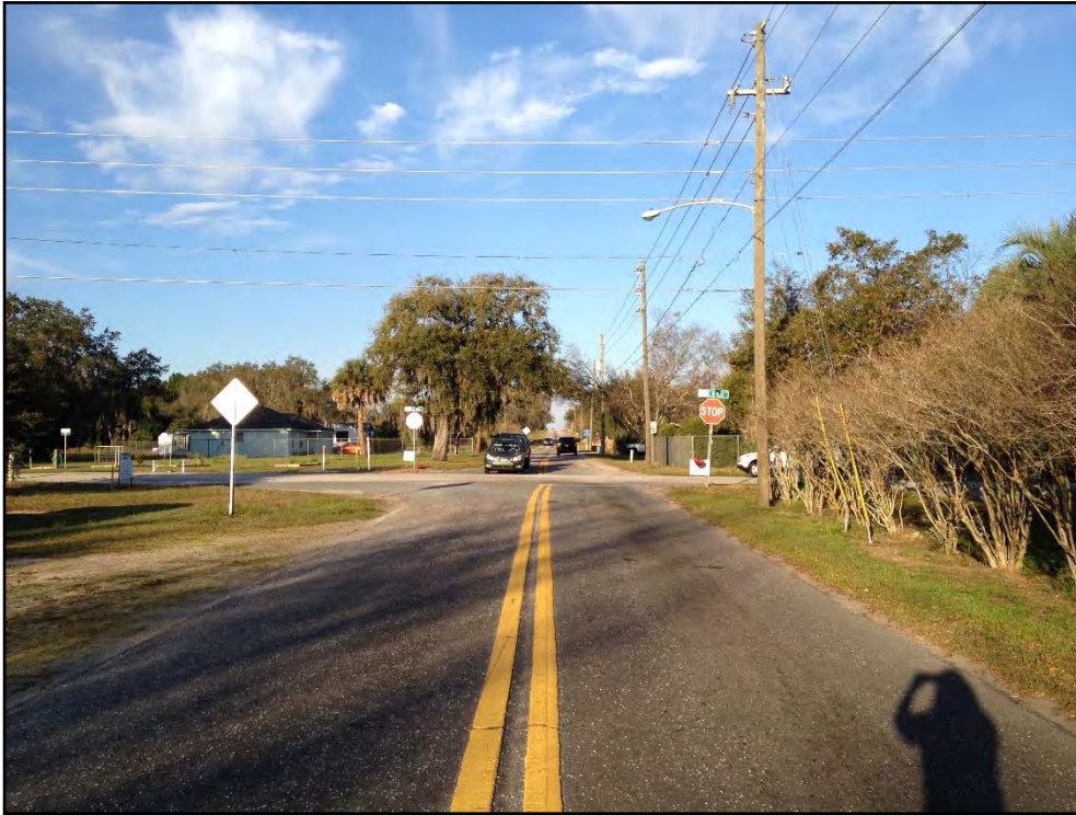
Exhibit 5: Looking west into the intersection along Ridgewood Avenue
