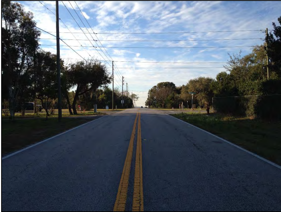
Exhibit 1: Looking south into the intersection along CR 455
