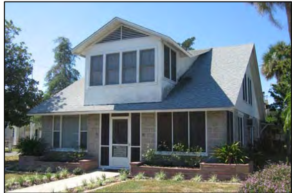
Figure 17. 8LA3443, Riley's Park Office. Photo facing west.
