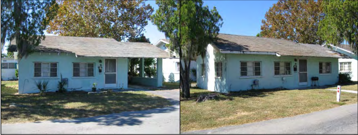
Figure 21. 8LA3456 (Cottage #18, left) is an example of a cottage with no alterations. 8LA3455 (Cottage #19, right) has several alterations including an enclosed carport, boxed eaves, and replacement of a portion of the original roofing material.
