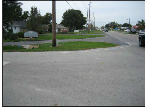
Figure 9. General Environment of the APE.
