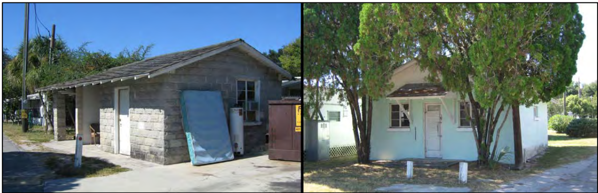
Figure 22. 8LA3500 (Auxiliary Bldg. #1, left) and 8LA3501 (Auxiliary Bldg. #2).
