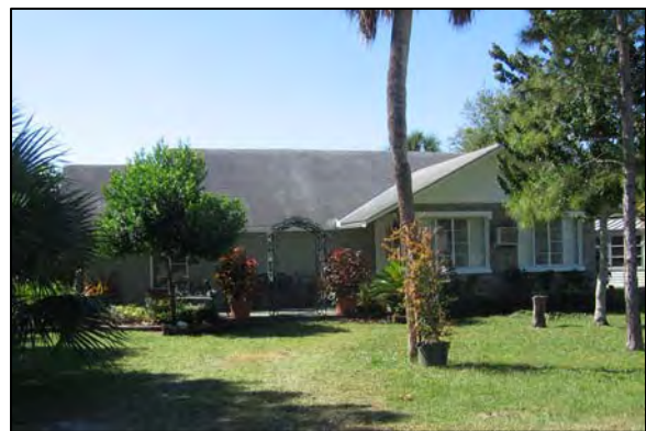
Figure 18. 8LA3447, Cottage #5, photo facing south.
