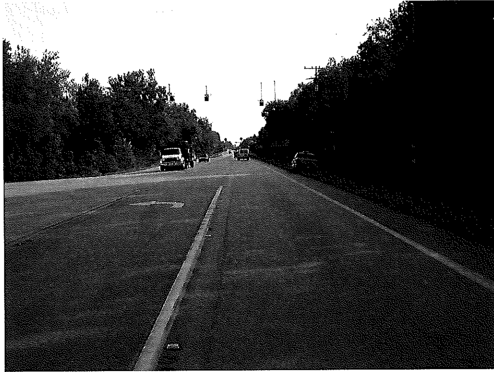
Looking east into the intersection along SR 44
