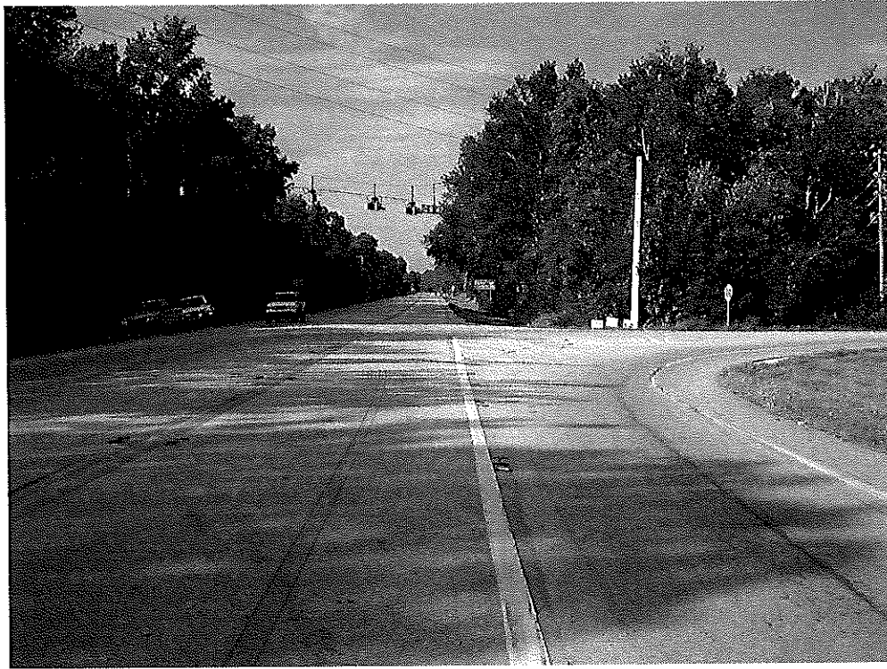
Looking west into the intersection along SR 44
