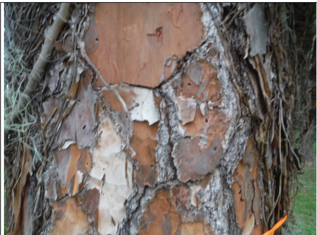
Minor Insect Boring Holes and Vine Roots Tree 2
