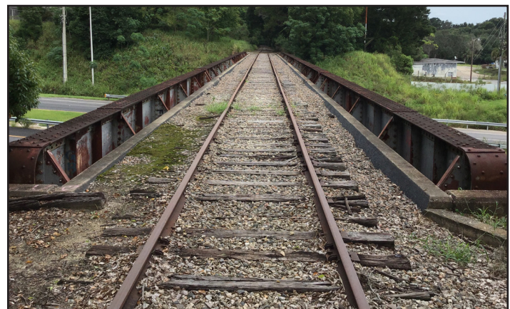
Existing steel bridge that crosses over US 441 (SR 500)
