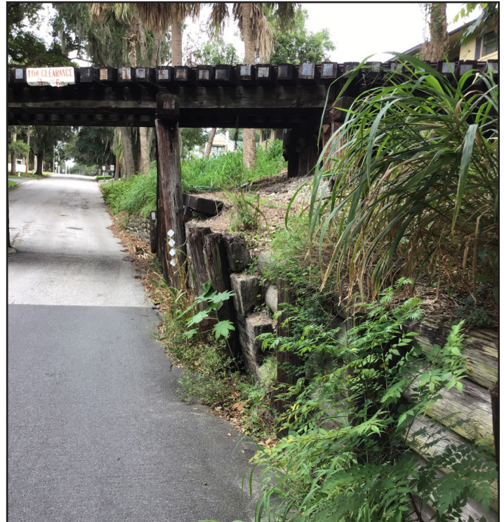
Relic Retaining Wall
