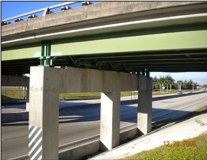
WGI's bridge jacking design over Florida's Turnpike
