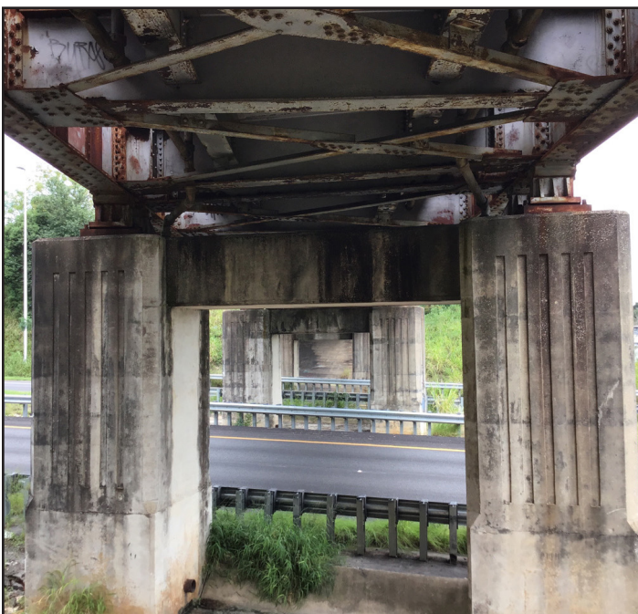
Existing bridge piers and supports over US 441 (SR 500)
