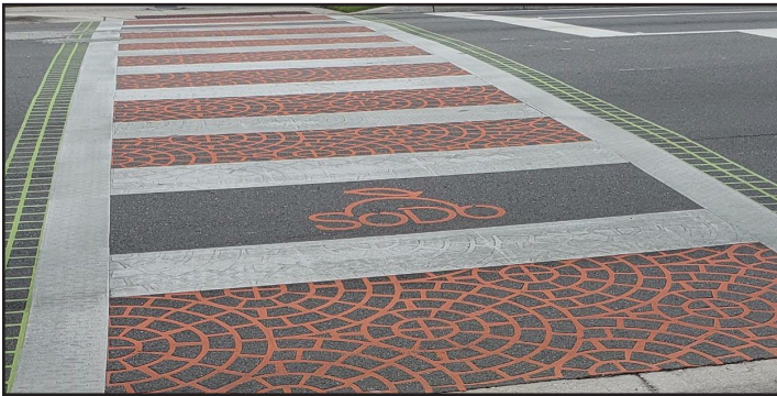
Patterned Crosswalks improve safety by providing a visual alert to motorists and pedestrians
