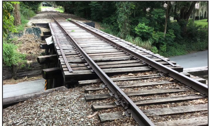
Existing timber bridge that crosses over Tremain Street
