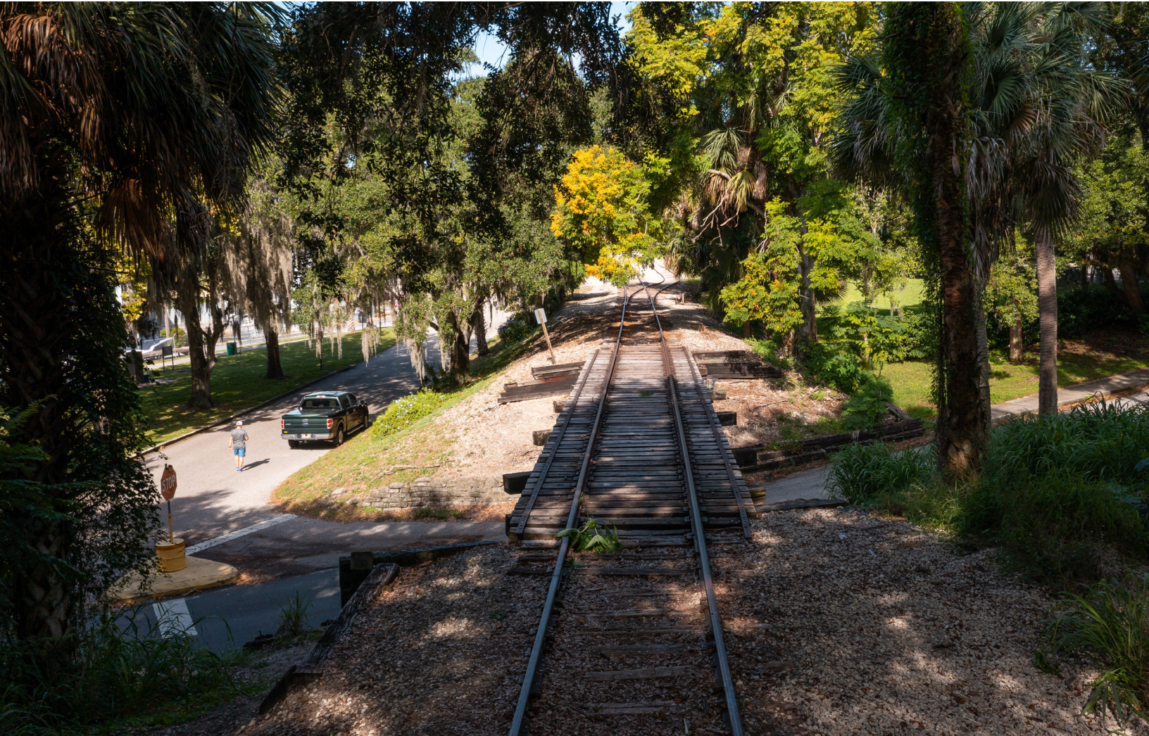
Tremain Street Bridge
