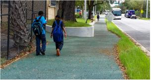
constructing the proposed path and curb and gutter and associated necessary modifications to existing drainage structures. The proposed 8 ft-10 ft-wide path utilized existing features of the roadway, including the alignment, impervious area, elevation, and existing drainage patterns. This project was designed to meet all rules and regulations set forth by SJRWMD, FDEP, and the City of Orlando.
