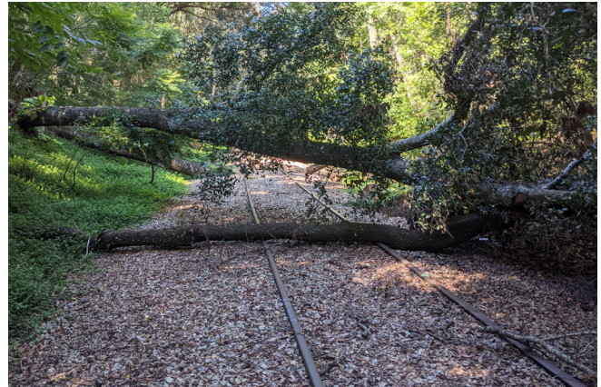
Tree Blocking Existing Rail Corridor
