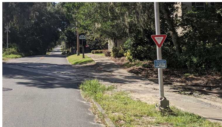
Sidewalk Connection at S. Clayton Street
