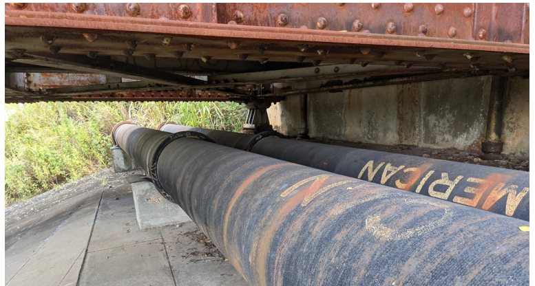
Sanitary Pipelines East Side of US 441 Bridge
