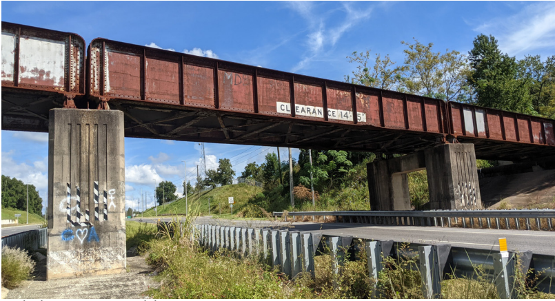
Existing US 441 Bridge
