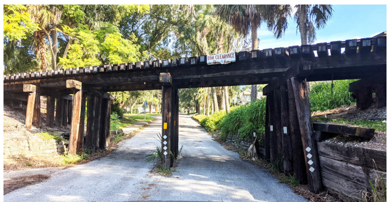
Existing Tremaine Street Bridge
