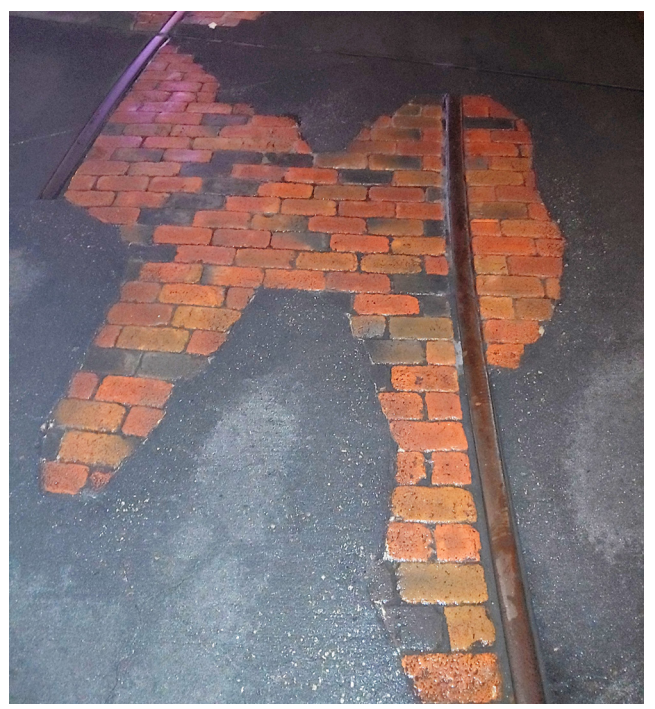
Photo Above: Rail historic preservation option (Design will ensure no tripping hazards exist)
