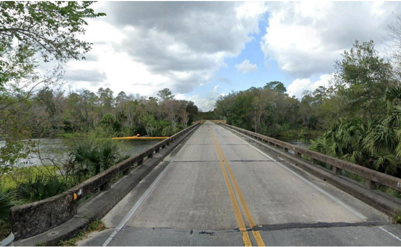
Figure 3-4: Bridge over Alexander Springs Creek looking south.
