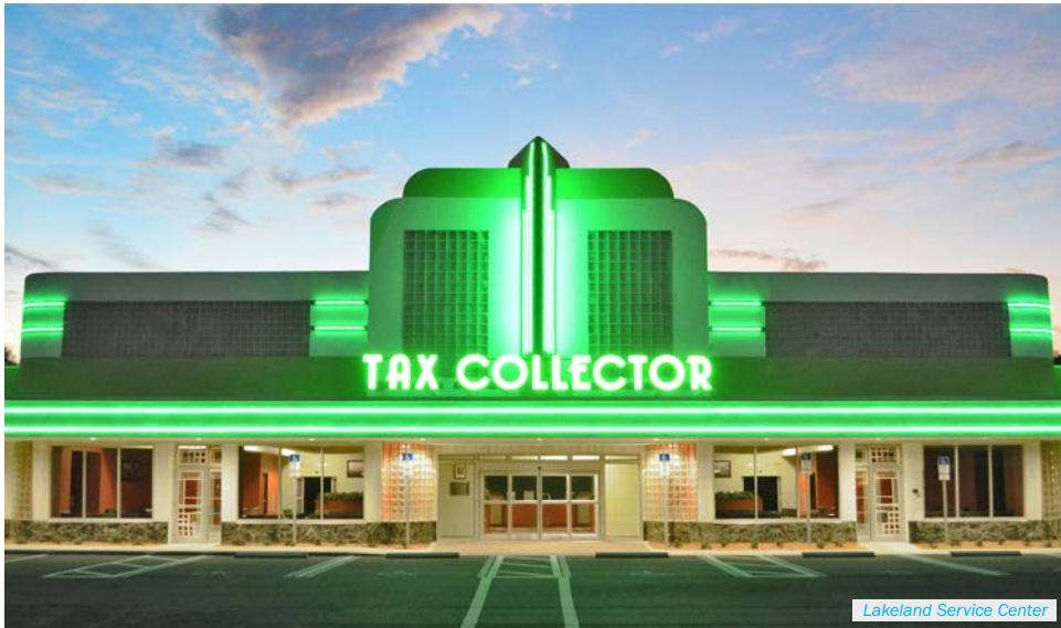
Lakeland Service Center
