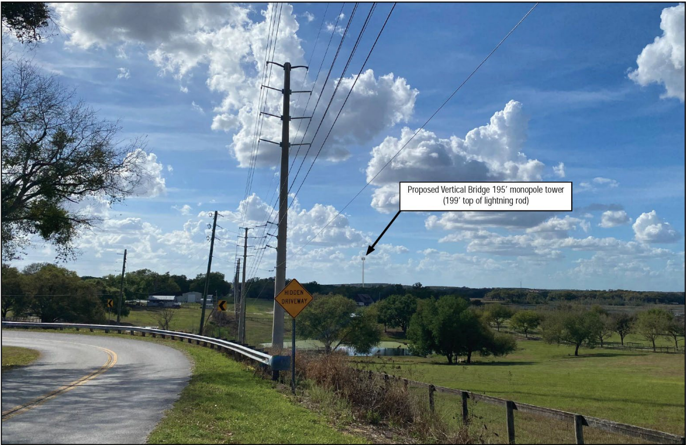
View #4 - Looking west from E Apshawa Road Proposed
