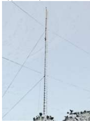
Typical Guyed Wire Tower
