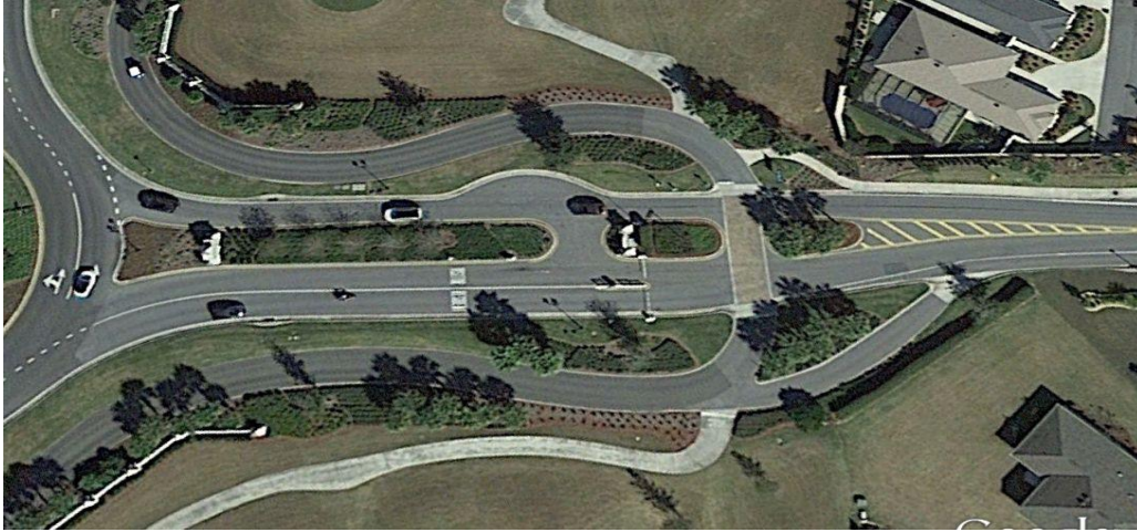
Figure 27: Typical unstaffed gate (no gatehouse)
