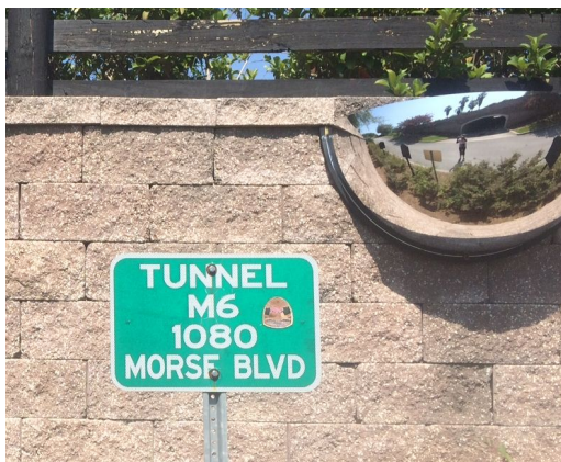
Figure 31: Tunnel identity sign (also note fisheye mirror)
