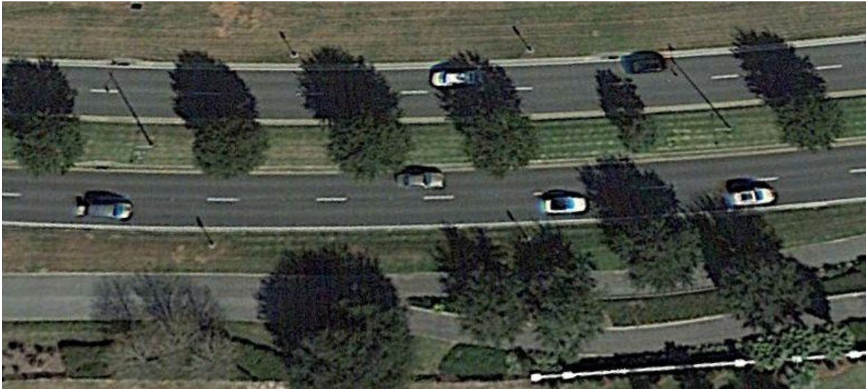
Figure 7: Arterial Road example: CR466 (45 mph), with 4 vehicle lanes, center island and parallel multi-modal path
