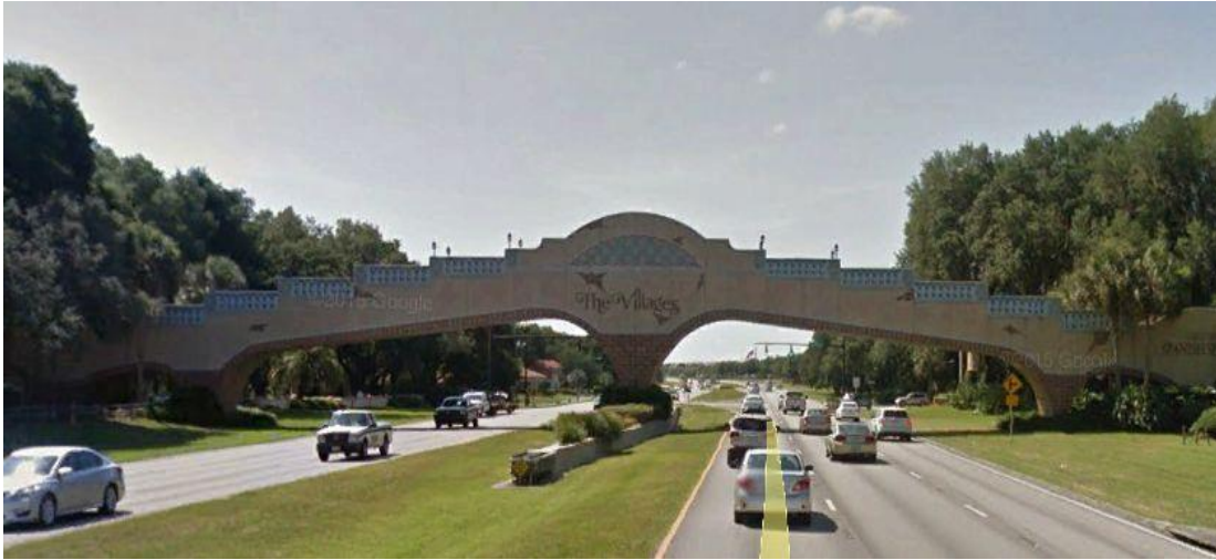
Figure 18: Multi-modal path bridge over SR 441/27
