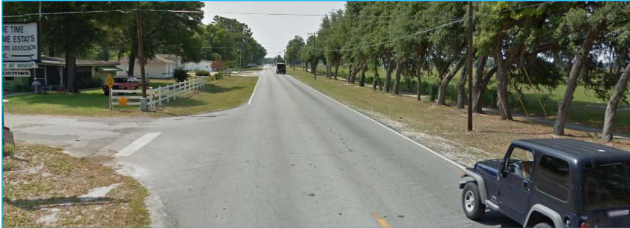
View looking south along CR 470 at the intersection with CR 461
