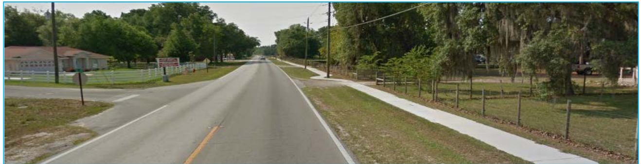
View looking south along CR 470 at the intersection with CR 486
