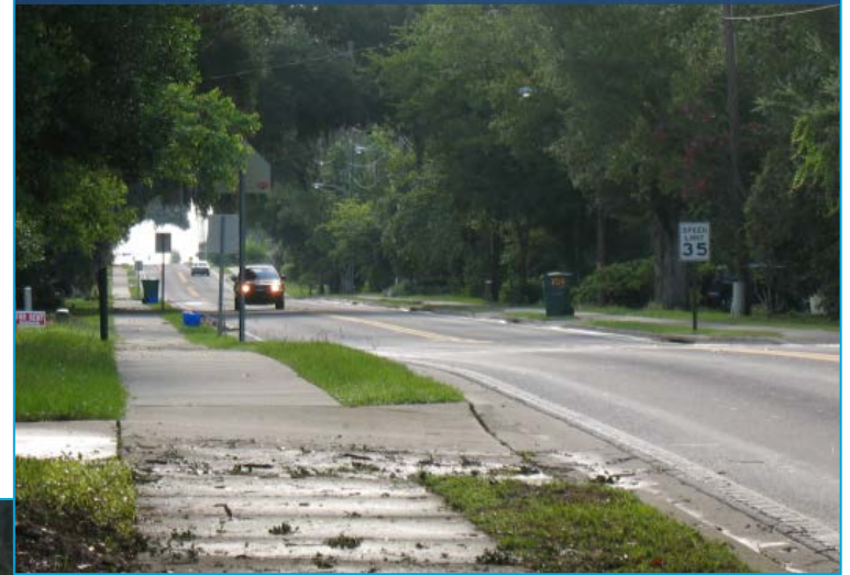
Cleveland Avenue looking east
