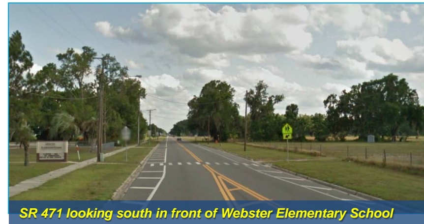
SR 471 looking south from S.E. 1st Avenue
