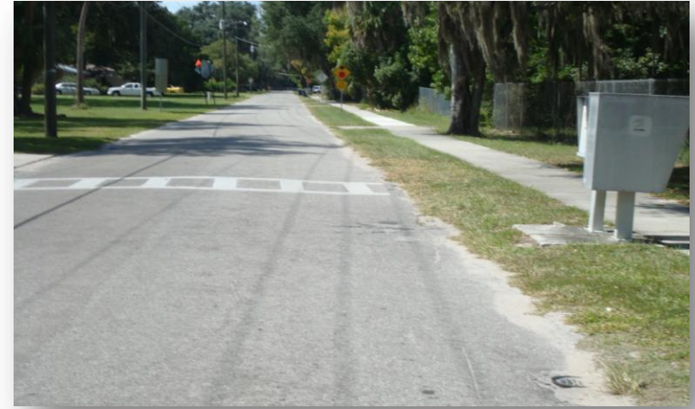
No sidewalk connection or signage currently available (W. Central Avenue looking west)
