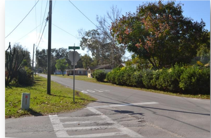
York Street and Central Ave – Crosswalk with no sidewalk connection
