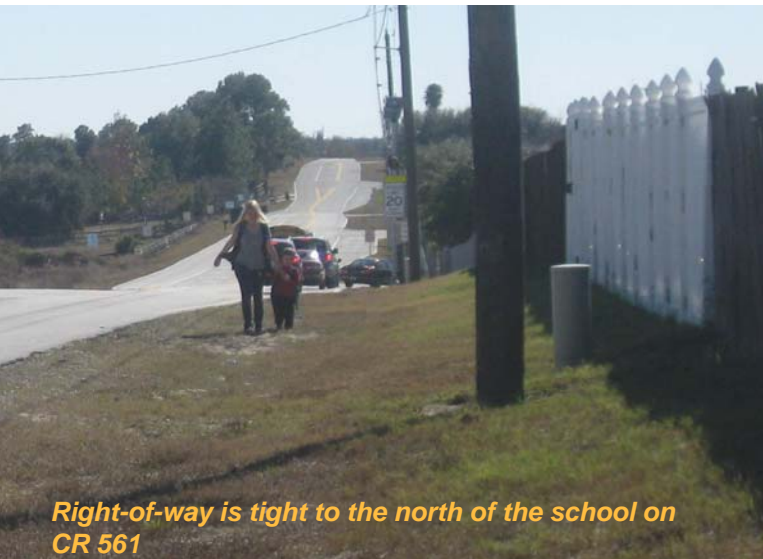
No sidewalks on CR 561 north of school
