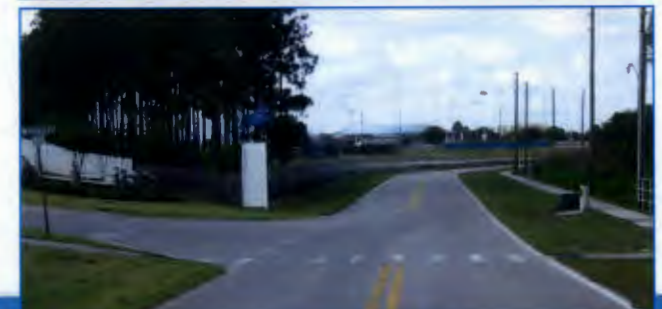
Maravilla Way crosswalk missing pedestrian signs
