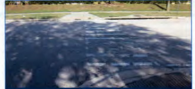
Existing Silver Eagle Rd Crosswalk at Senior Lot
