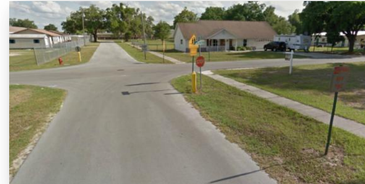
The intersection of S.E. 1 st Street and S.E. 1 st Avenue lacks stop bars and crosswalks
