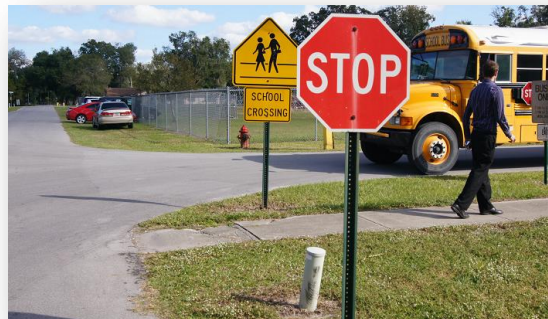
The stop sign is mounted too low at the intersection of S.E. 1 st Street and S.E. 1 st Avenue
