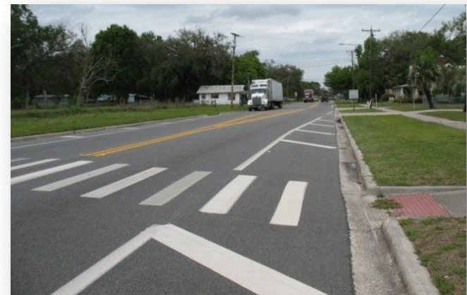
SR 471 – Webster Elementary School crosswalk
