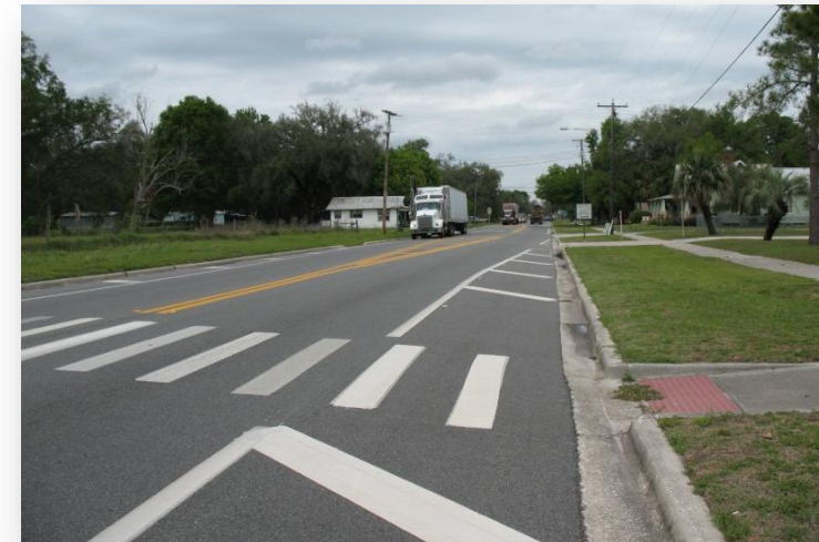
An unstaffed crosswalk is located in front of the school
