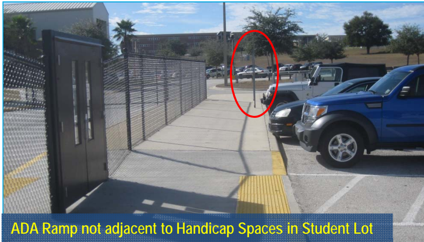
ADA Ramp not adjacent to Handicap Spaces in Student Lot
